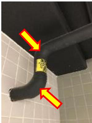
Photo 1: Asbestos-containing parging cement insulation on pipe elbows – Men's Washroom.
