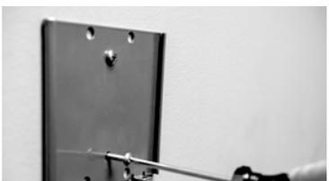
Eyeball the halfway point between the screwholes **d** on **K**. Don't worry about making it level at this point. You will just need to establish the first hole on the upper portion of **K** and mark it with the pencil. It is essential to keep the wider part of **K** at the top and the two Security Screw hole extensions (**e**) on the bottom.
