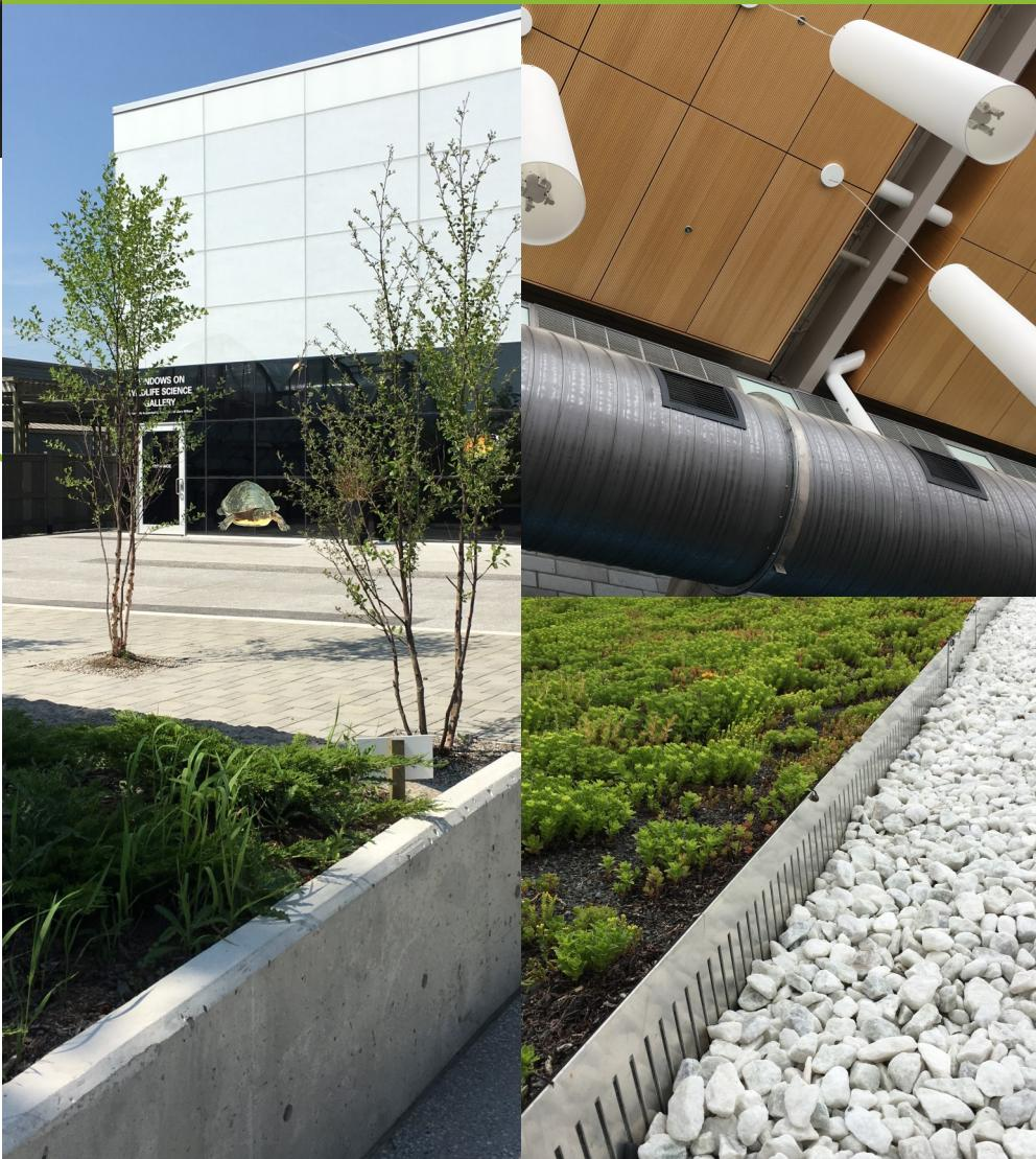
A green roof spanning 5,200 ft<sup>2</sup> covers most of the roof area, with the rest being an energy-efficient white roof. This is one of four green roofs at the Zoo, spanning a total of 12,673 ft<sup>2</sup>. The building has a double foundation wall constructed with continuous insulation sandwiched between the walls, reducing heat loss. All washroom fixtures have a "low-flow" design.
