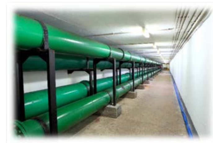
Underground pipes carrying water for cooling
