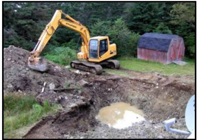
Pond construction © John O'Connor
